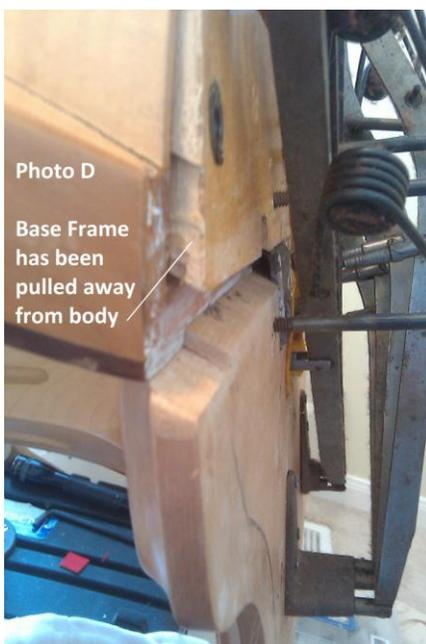
Photo D shows what can eventually happen if this situation is not corrected. Here, the baseboard has been pulled way out of alignment with the body, and it has dragged the base frame along with it. This harp's regulation is likely to be severely compromised. In addition, it will be off balance, and will tend to tip backwards much more easily than it should, leaving it open to further injury.
